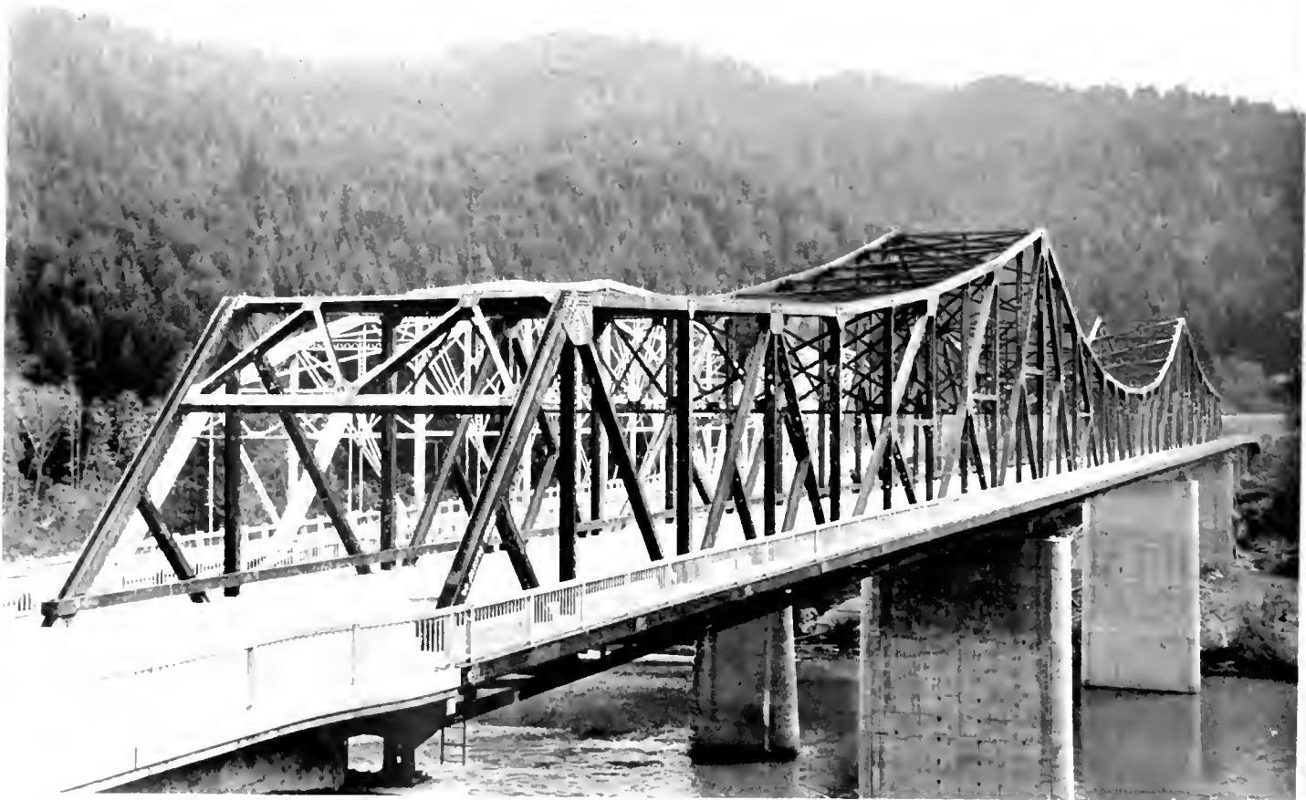
New North Scotia Bridge which supplants old span on the left that has been condemned as unsafe by Division of Highways
